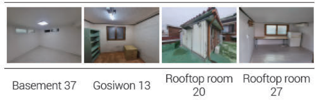
Figure 5. Examples of uninstalled residential fire facilities
