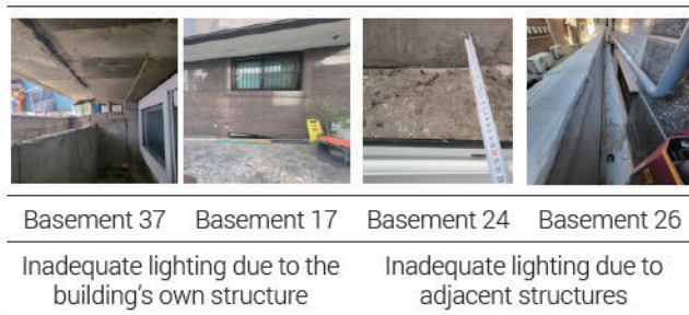
Figure 2. Examples of window structure that influenced natural lighting
