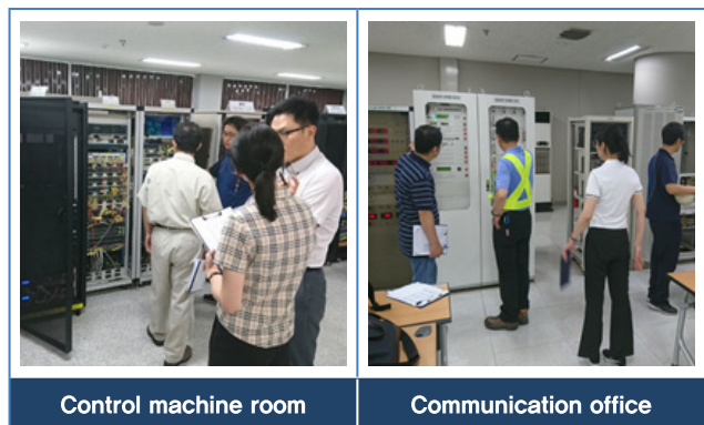
Figure 2. Field investigation photos
